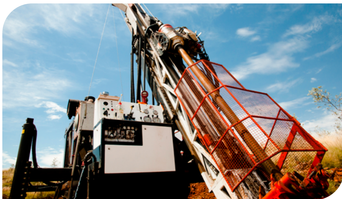
Core drilling provides physical rock samples that can help characterize subsurface geology.
