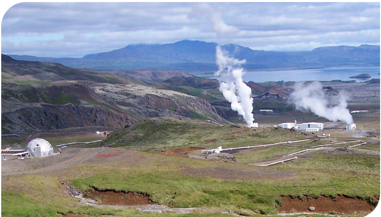
Geothermal generation plant in Iceland.
