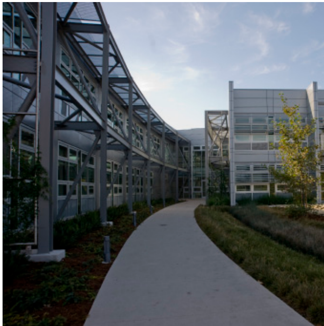
FIGURE 1: Groundlevel View of Sustainability Base
