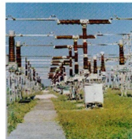
Live tank breaker (Courtesy BHEL)
