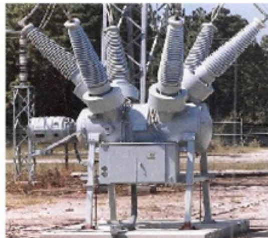
Dead tank breaker (courtesy ABB)
